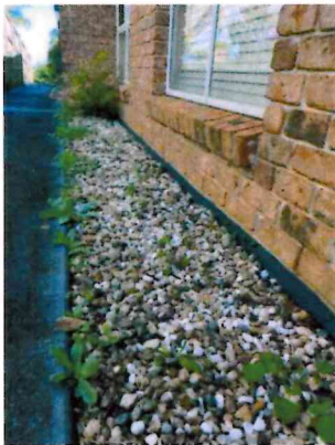
Showing exposed slab edge.
