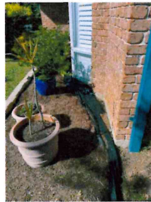
Showing newly exposed slab edge in front garden.
