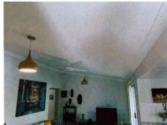
Showing internal roof structure.
